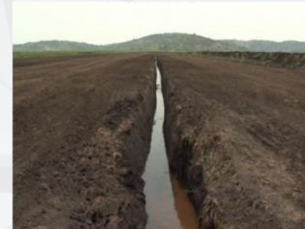
Secondary ditches (1.5m deep)
